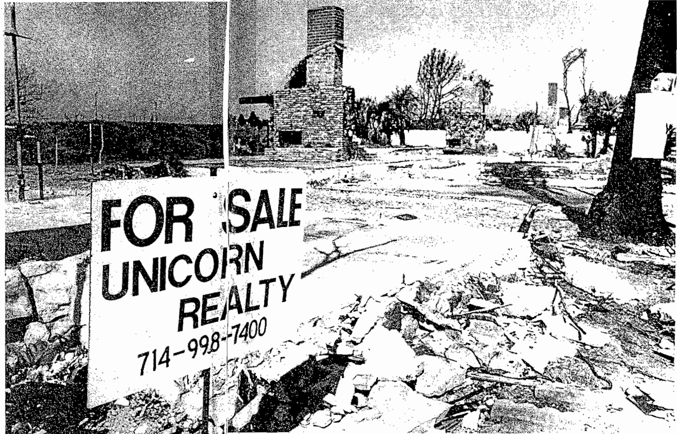
A 'for sale' sign is the only recent addition to this property which was devastated by an arson fire on July 2. The fire destroyed or damaged 66 homes.
